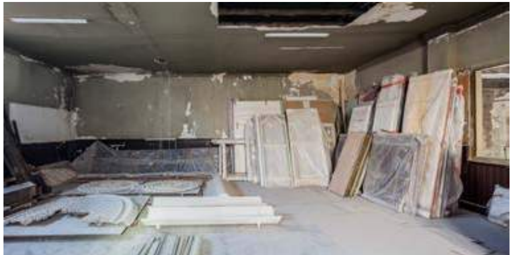
1. The Sala Beckett in Poblenou during reform work © Adrià Goula.
